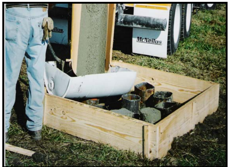
Concrete pad poured over the CHPP piles
