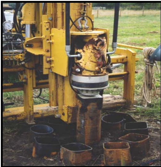
Cluster of CHPP helical piles installed for the Tower foundation
