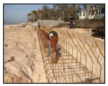
Lightweight maneuverable equipment with a hydraulic torque motor was used to install the CHPP helical piles
