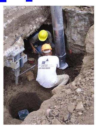
The formed square connection ends transfers installing torque through the pipe pile and not through the bolts
