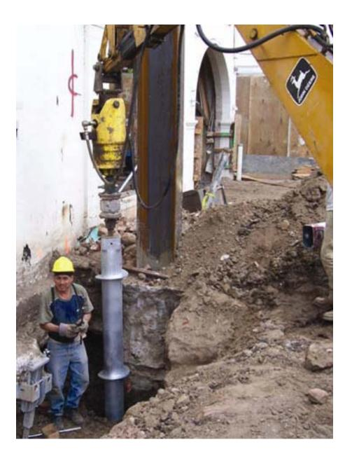
Lightweight and maneuverable equipment was used to install the helical piles.
