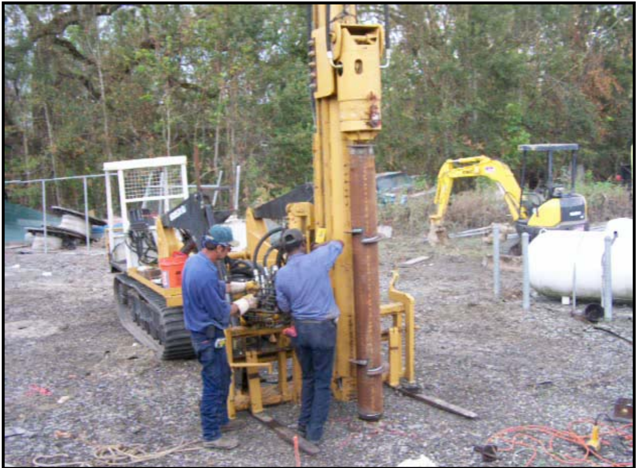
Lightweight and maneuverable equipment installed the helical piles on this project
