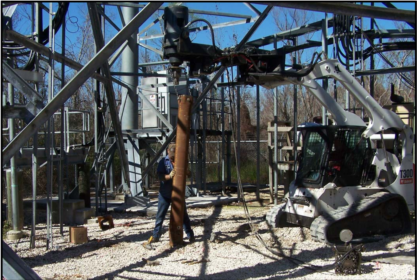
Lightweight and maneuverable equipment was used to install the helical piles
