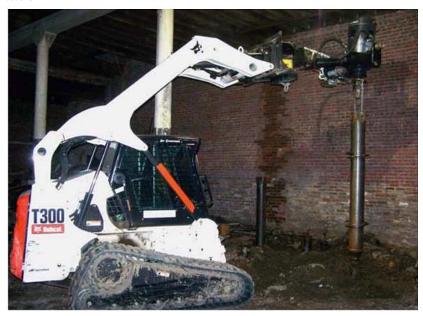
Lightweight and maneuverable equipment was used to install the helical piles
