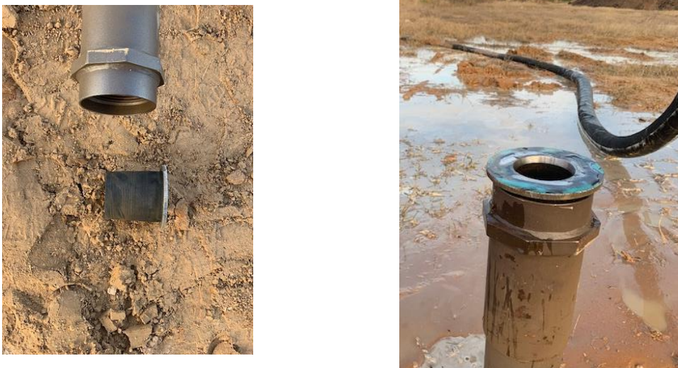
Figure 1: Typical grout plug shown on the ground and in a threaded coupling
