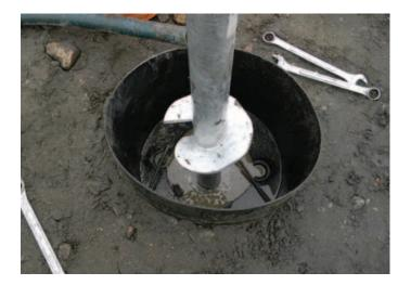
STEP 1: Insert the Helical Pile Lead
