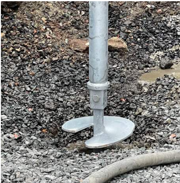
Seamlessly couple square bar leads to pipe extensions.
