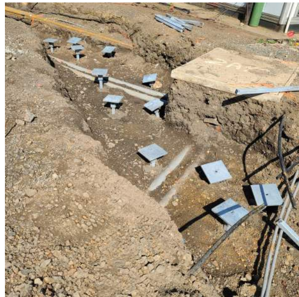
Battered piles with termination brackets installed adjacent to an existing pipe.
