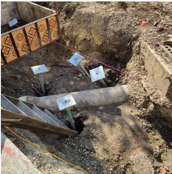
Battered piles with termination brackets installed adjacent to an existing pipe.
