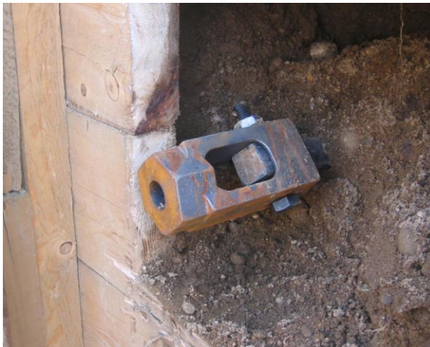
Tieback adapter for RCS helical tieback anchors and Williams threaded rebar
