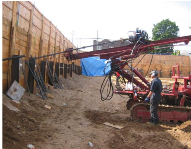
Installing Round Corner Square (RCS) helical tieback anchors
