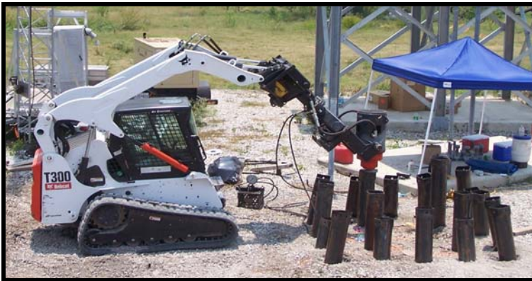
Lightweight and maneuverable equipment installed helical piles
