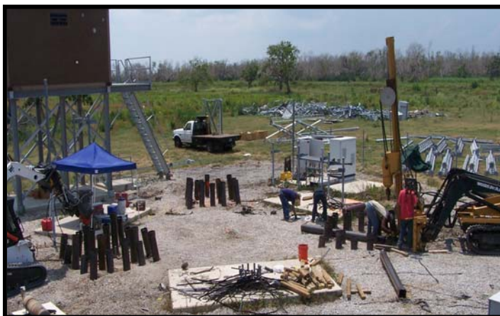
The three CHPP helical piles installed
