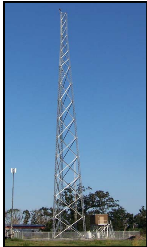
New tower installed on the 60 CHPP helical piles
